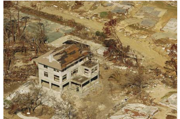
This ICF house was a lone survivor after the storm surge from Hurricane Katrina in 2006.
